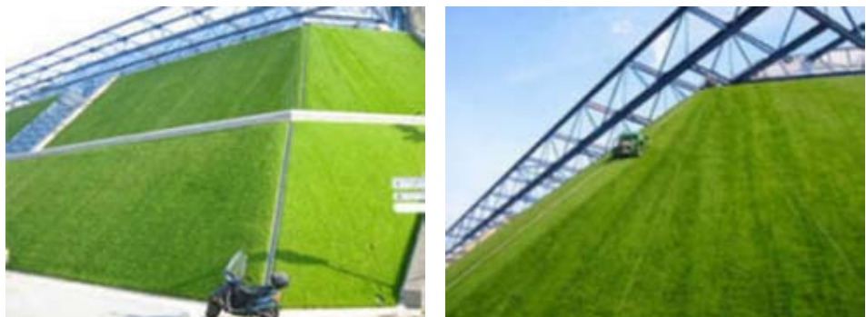
Ford Motor Plant – Dearborn, Michigan. The biggest green roof in the world at 10.4 acres
