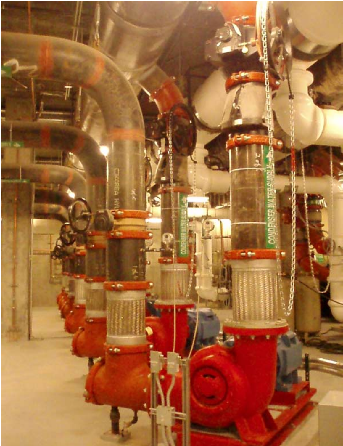
Southland Industries Pipe Fitting Chiller Room project
