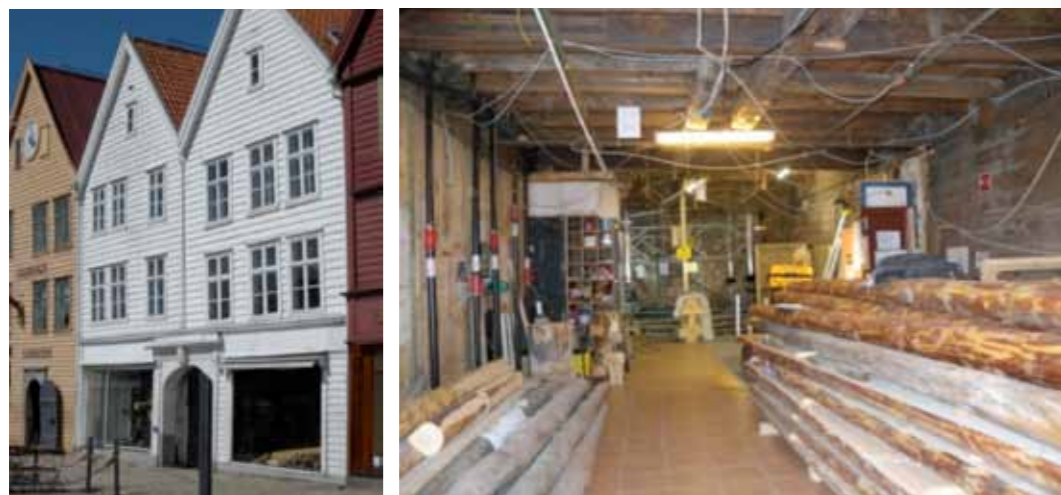
Left and right: An old warehouse by the wharf undergoing restoration, Bryggen World Heritage Site, Bergen
