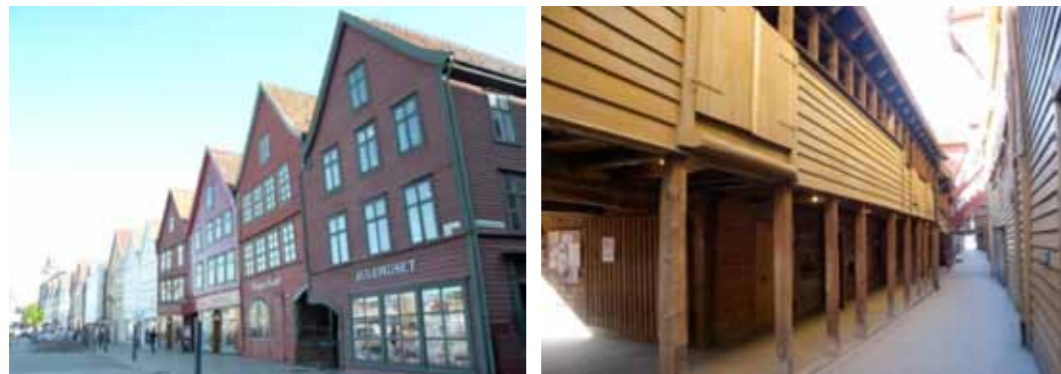
Left and right: An old warehouse by the wharf undergoing restoration, Bryggen World Heritage Site, Bergen
