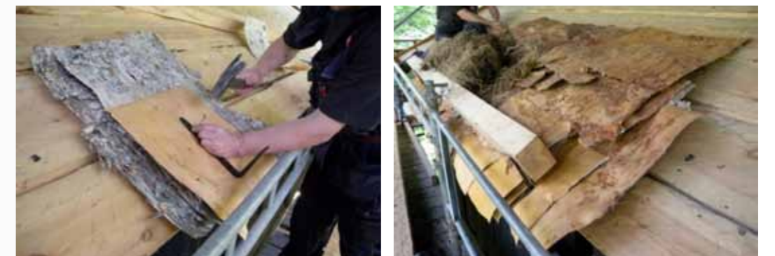
Laying a birch bark roof over a planked roof
