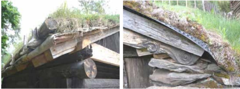
A traditional birch bark roof, consisting of layers of overlapping birch bark as waterproofing, with soil above for insulation
