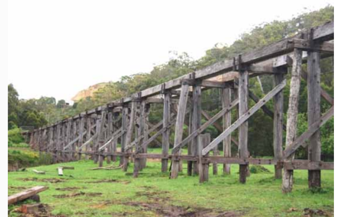
Curdies River Bridge, Timboon, Victoria
