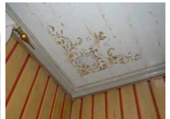
Conservators from the local museum were consulted to assist in recovering the original stencilling
