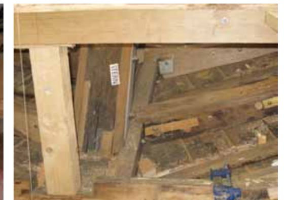
Inside the hull near the stern showing new stainless steel fixtures and fittings
