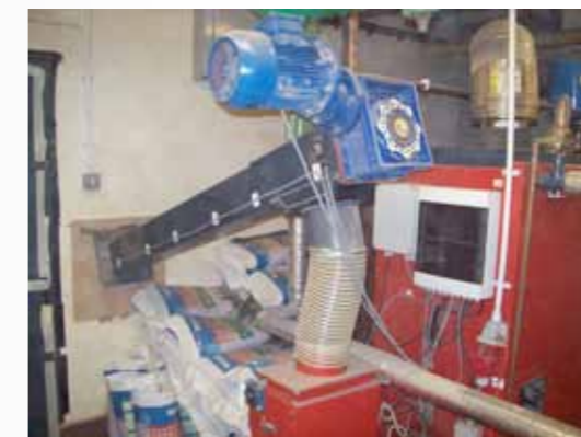
Figure 30: Feed auger for pellets from old coal store in basement of school (also pictured are some spare bags of pellets)
