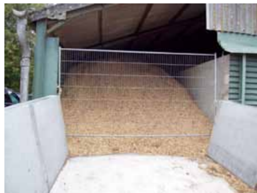
Figure 39: The outside view of the wood chip storage bay (note the accessibility for tractors or loaders to deliver chips into the storage unit)
