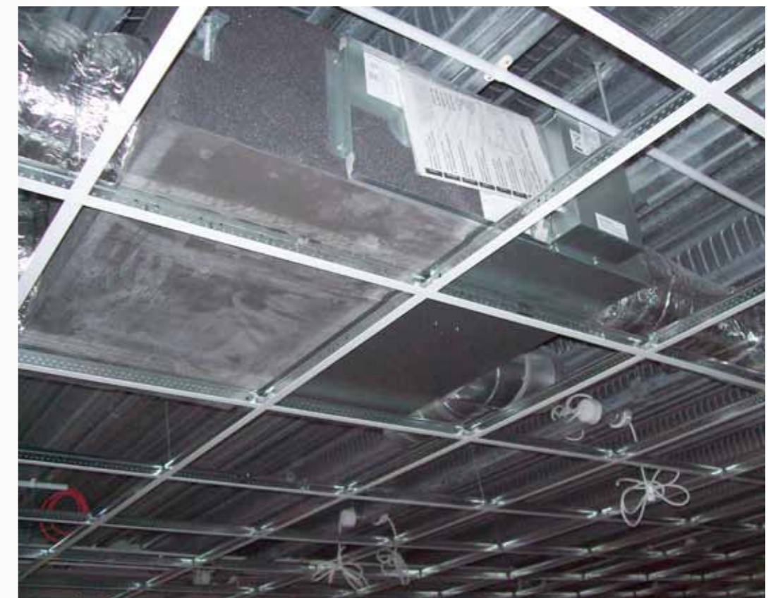
Figure 9: The air handle unit in the ceiling area of a crèche on the ground floor building of Údarás Industrial Park
