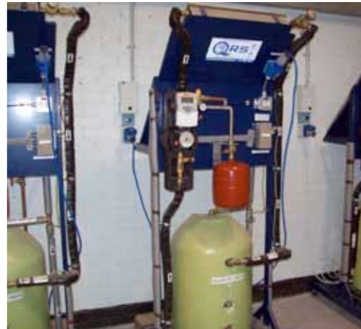
Figure 14: Mobile solar hot water training workstations at FAS
