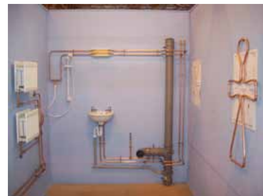
Figure 50: Some of the work done by the award winning plumbing apprentices
