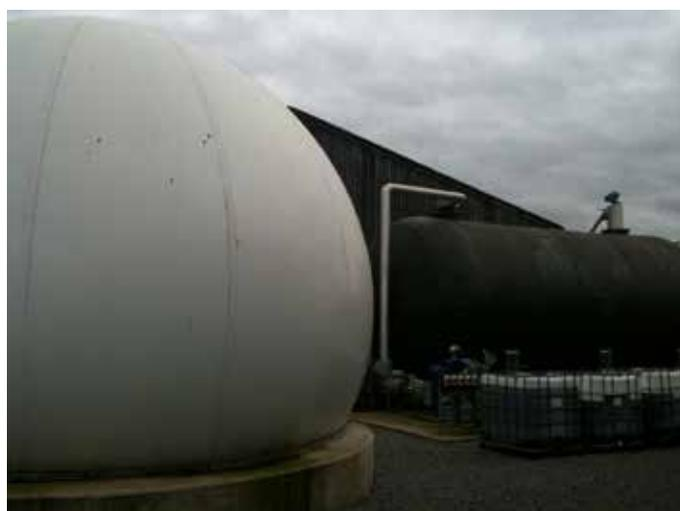
Figures 9, 10 & 11: Reaseheath College Bioreactor (anaerobic digestion plant) generating power and heat from a range of farm effluent streams (shown in Figure 9); a reactor chamber and the gas storage cylinder in Figures 10 and 11 respectively. Operational challenges have been experienced that strongly indicate that on-going support and training are critical to smooth integration.
