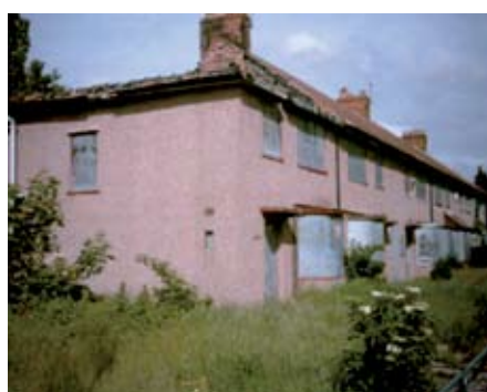
Boswell houses on the Boot Estate awaiting demolition
