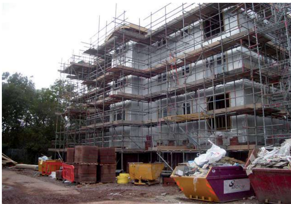
Colour-coded waste bins
