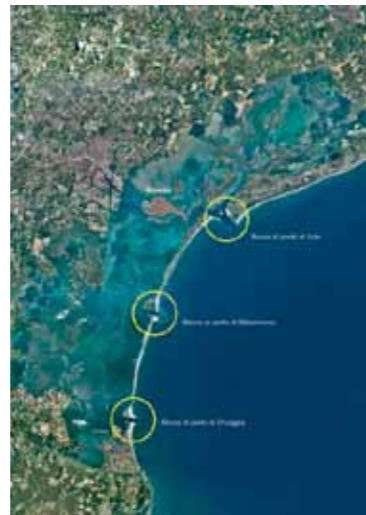
The three inlets where the MOSE Project gates will be positioned
