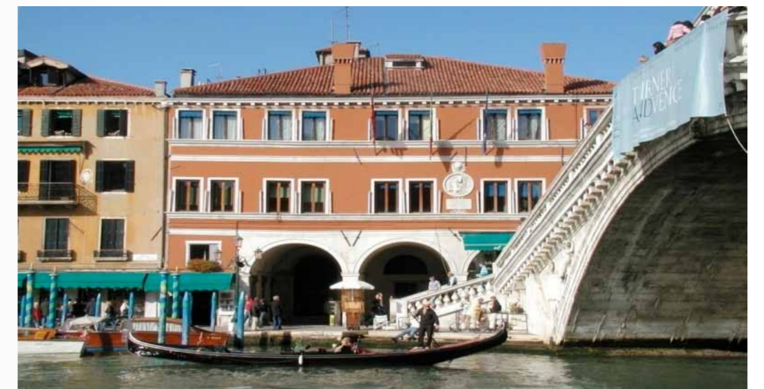
The Venice Water Authority near the Rialto Bridge
