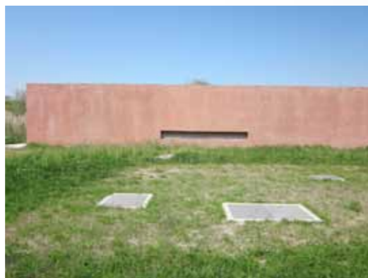
The integrity of the landscape is maintained with treatment basins below ground
