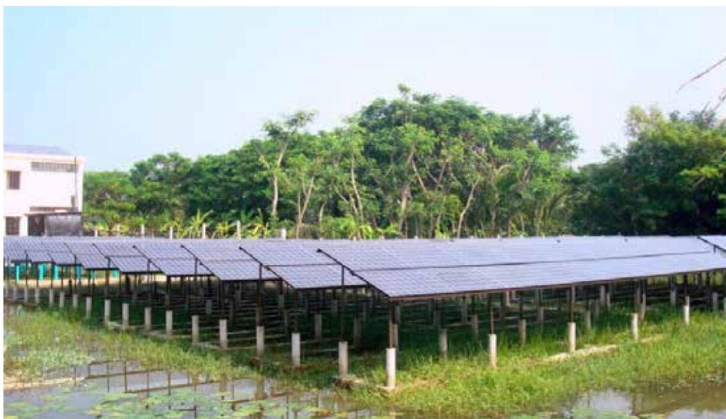
Figure 13. The 100 kW solar minigrid on Sandwip Island, Bangladesh – standalone (off-grid) project that has provided energy access to this remote community using innovative project design (Image: Ahsanul Hoque).
