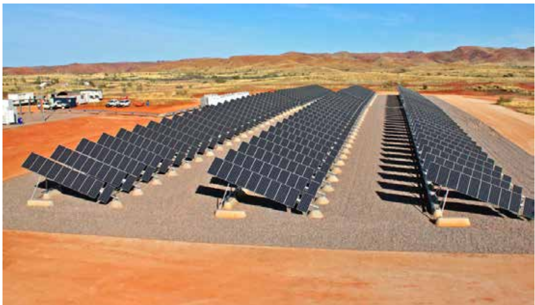
Figure 5. Horizon Power's Pippunyah power station in Marble Bar (Western Australia), which combines a single axis tracking 1.16 MW solar farm with diesel generation and kinetic flywheel energy storage. 8
