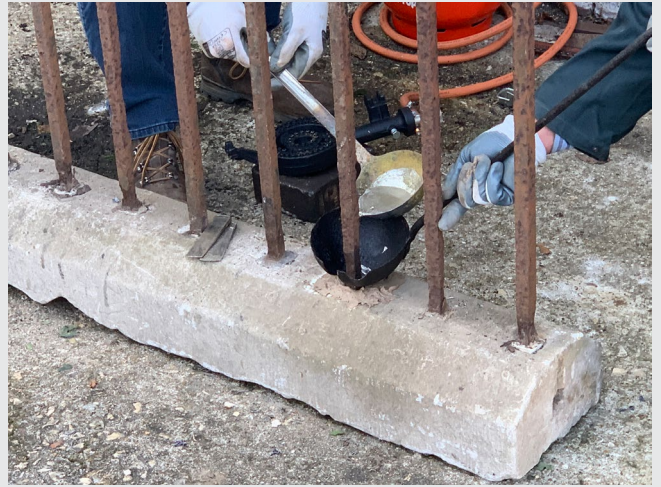
The molten lead is carefully poured into the void below the railings.
