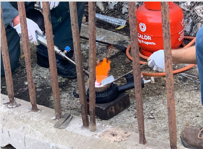
To reinstate, firstly lead is melted in an iron crucible using an oxy torch.
