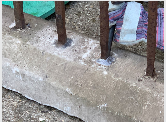
The lead is shaped using hammers and cold chisels to refine its form.
