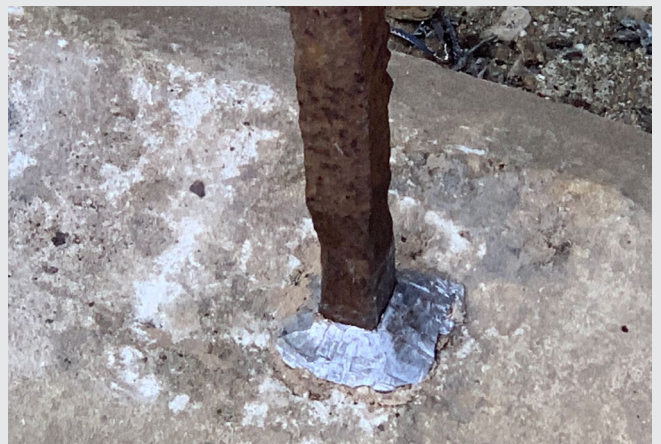
The finished reinstallation of the iron railing.
