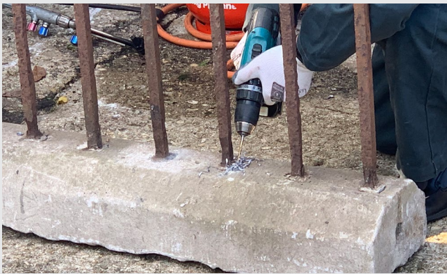
This photo shows the removal process, Geoffrey is drilling a series of small holes around the railings, before using plyers and lever bars to remove the individual railings
