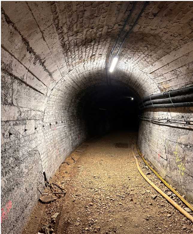
Figure 8. One of the original iron ore mine tunnels at ZAB, Eisenerz, Stryia, Austria
