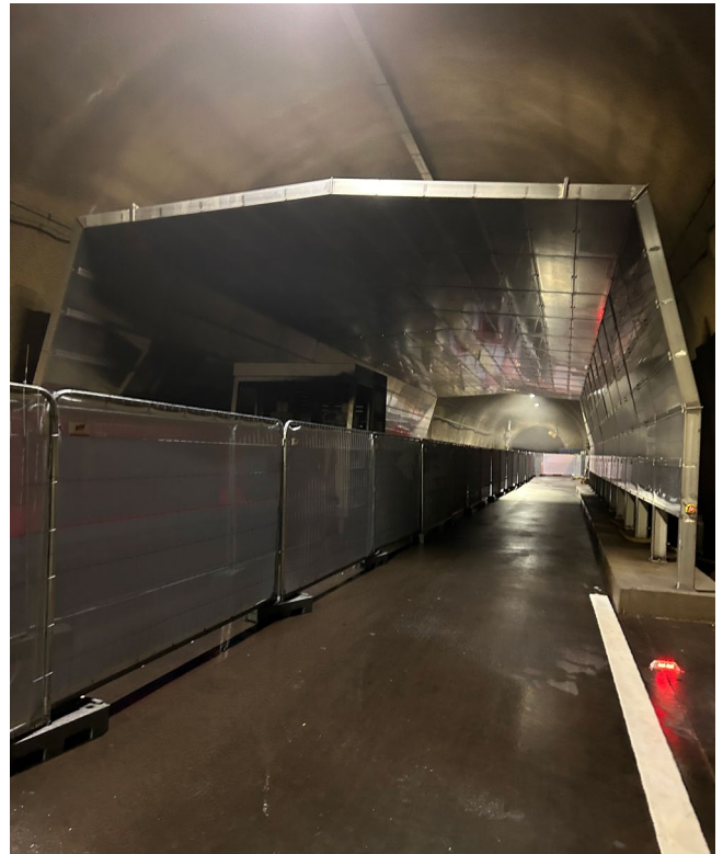
Figure 9. Heat shield in two lane road tunnel at ZAB, Eisenerz, Stryia, Austria
