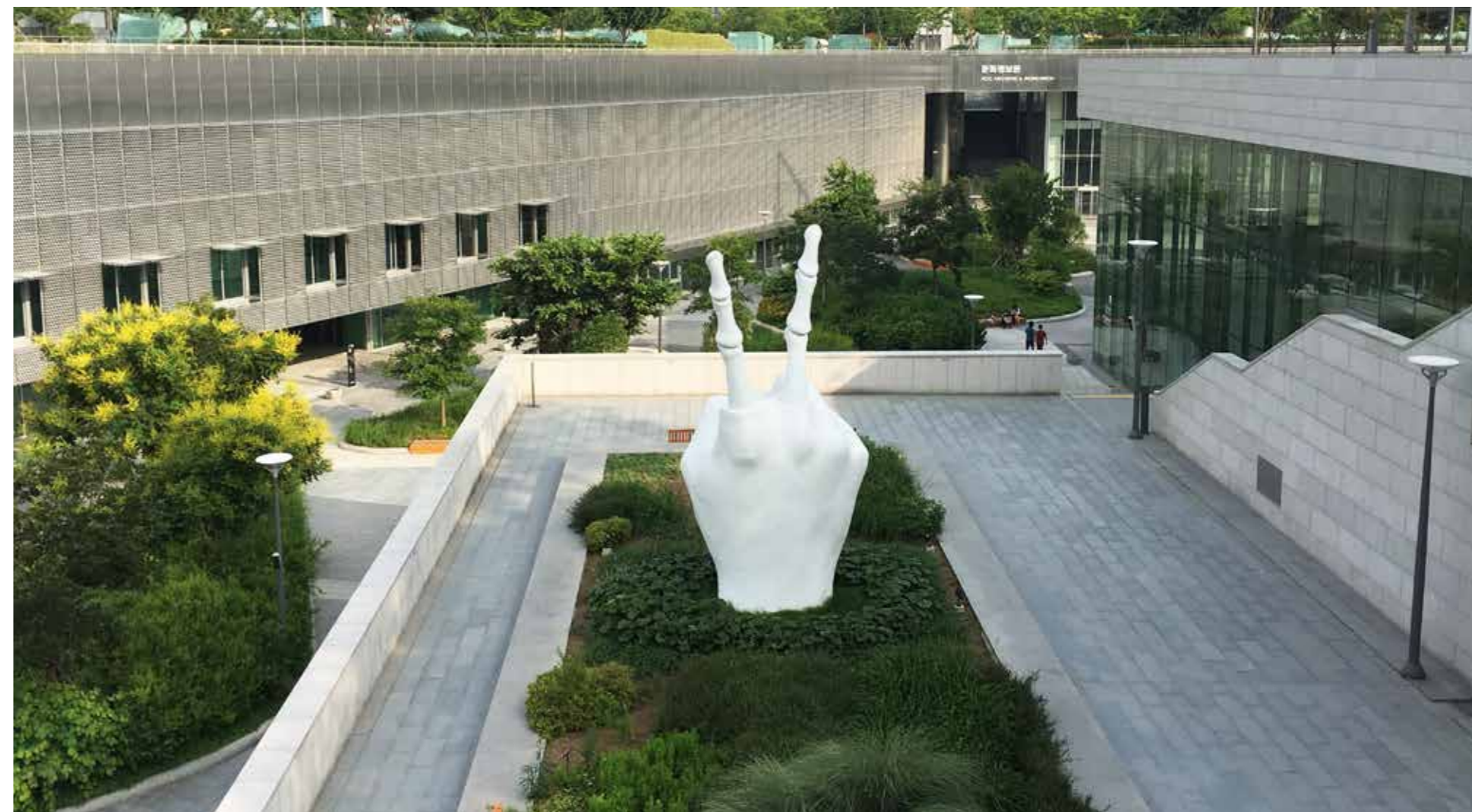
Looking down into the excavated site of the Asia Culture Center, Gwangju, South Korea
