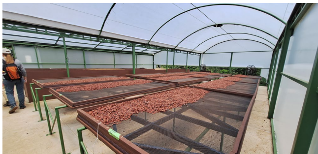
Figure 19. Drying shed and tables
