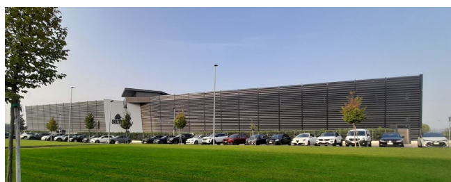
Figure 55. SELMI Head office and factory, Pollenzo Bra Italy
