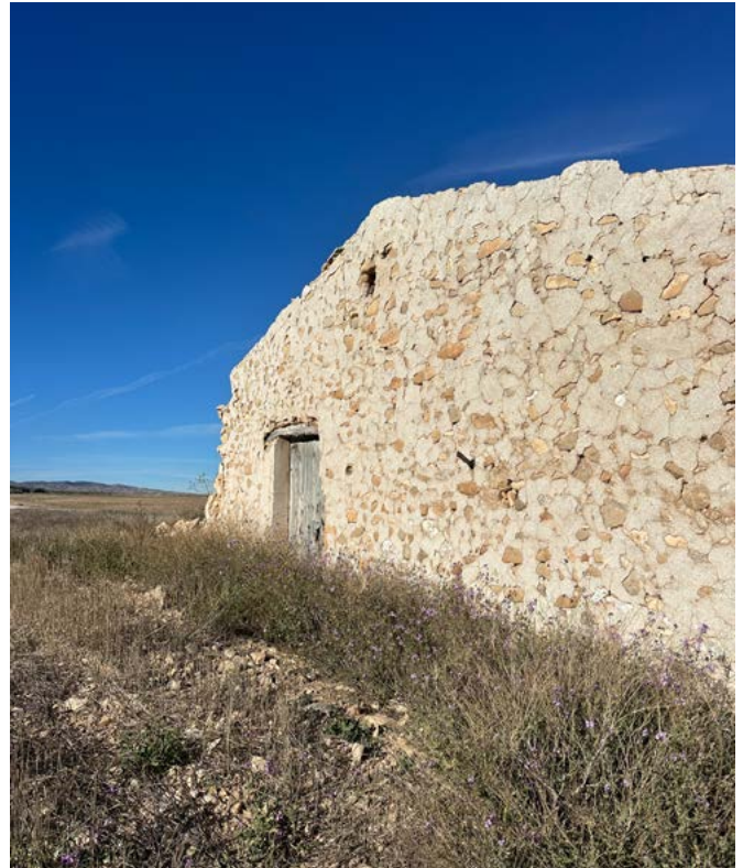
Figure 34. Nineteenth-century house constructed from alabaster stone, with ground gypsum used as mortar. Image credit: Marlo Lyda.
