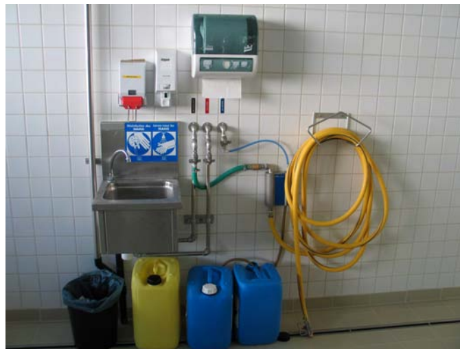
The ideal wash and sanitizing station. Soap, paper towel, hot, cold, high pressure tap, sensory wash trough and rubbish bin.
