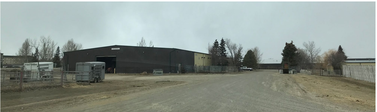
Figure 44. Olds College Rodeo training facility
