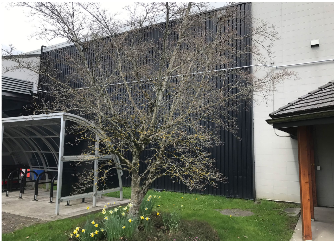
Figure 32. Camosun College Plumbing Centre solar wall
