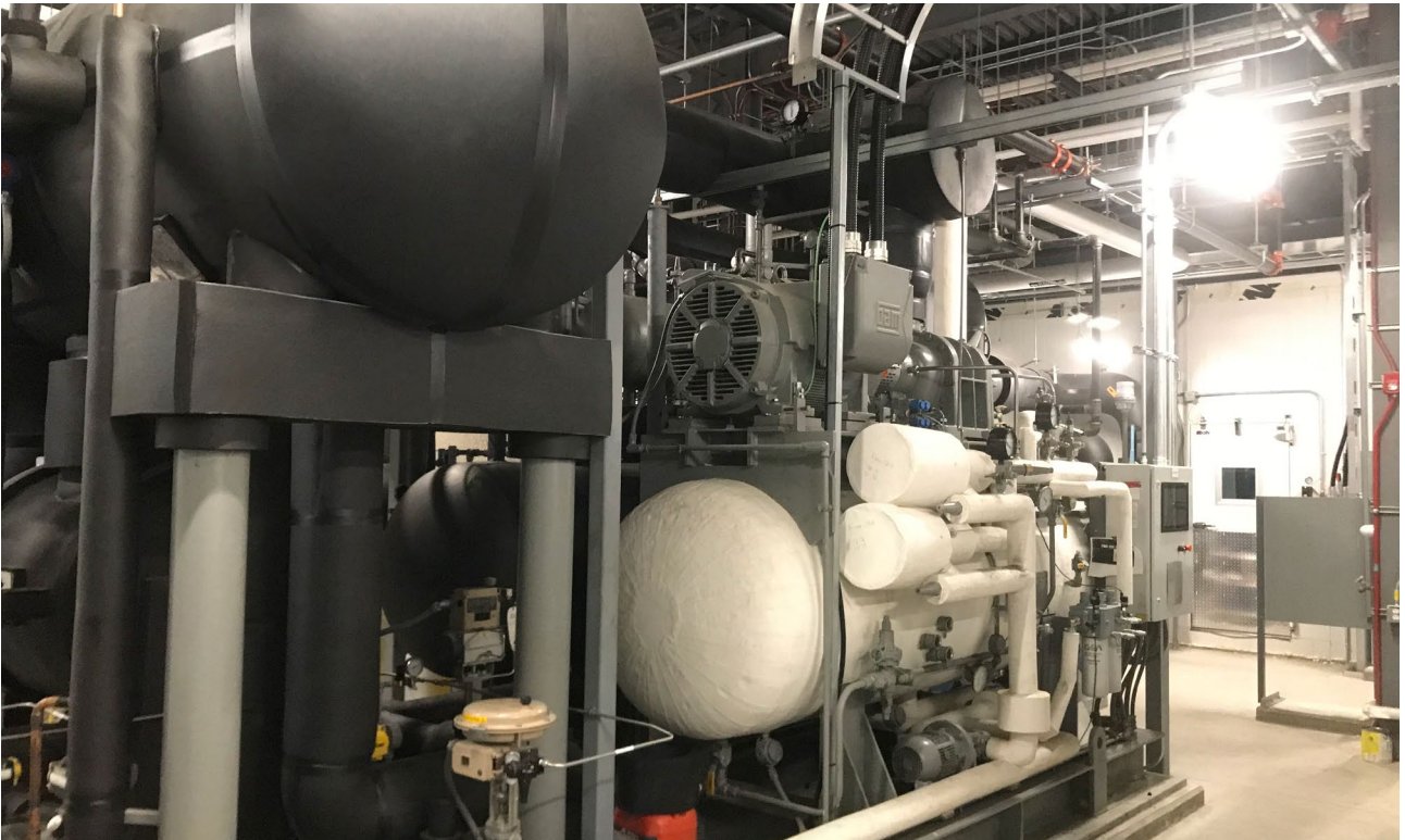
Figure 59. RRC Dynot lab -40C to 40C, 6kL coolant system
