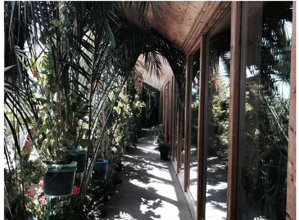
Greenhouses within the buildings at the Earthship Academy keep interior spaces cool by evaporative cooling of the space.
