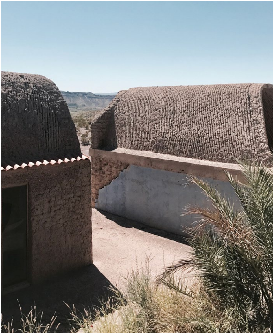
Adobe brick vaults made from local materials at the Simone Swan house in Presidio Texas.
