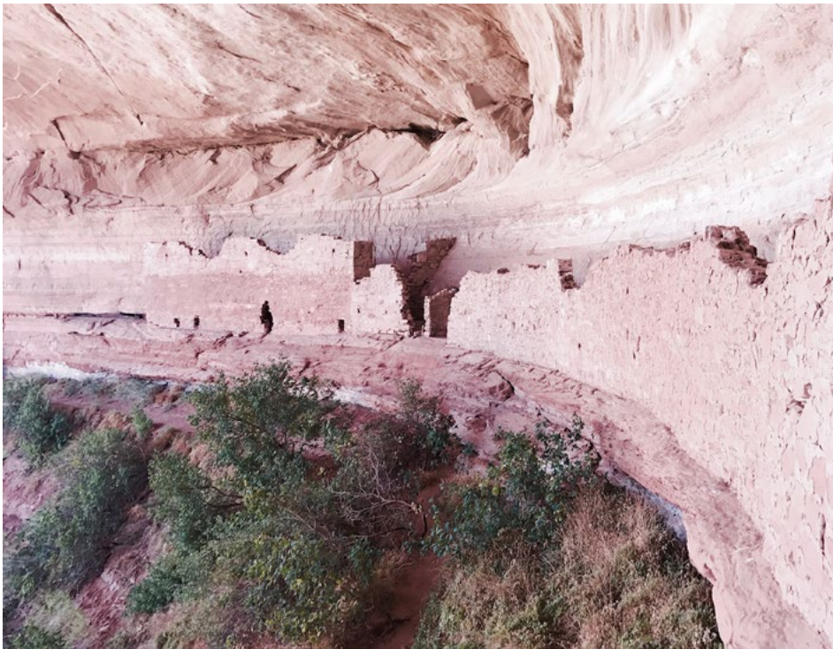
Ancient Cliff Dwellings in Utah made from rock masonry and mud mortar.
