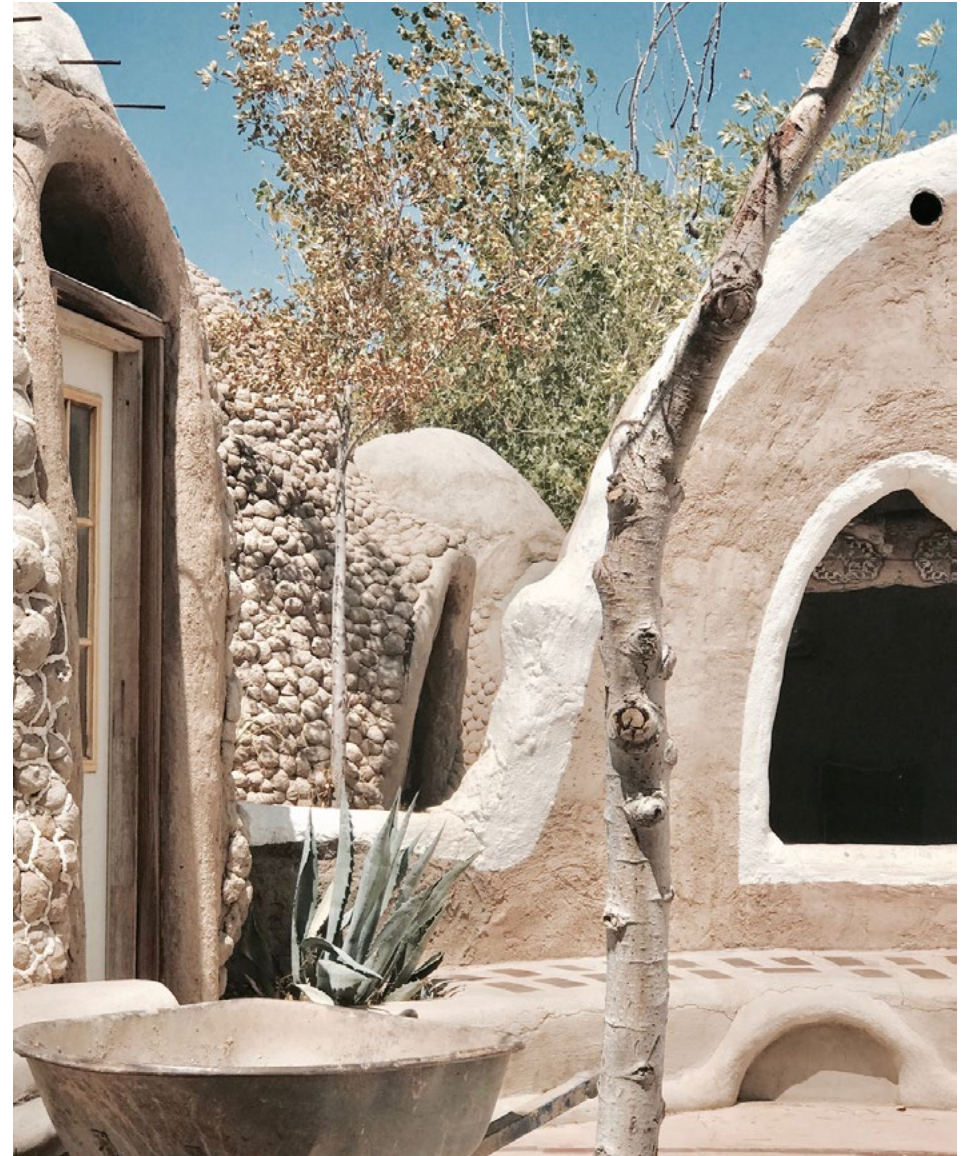
At Cal Earth each building is customised using earth and wall paints made from local clay.
