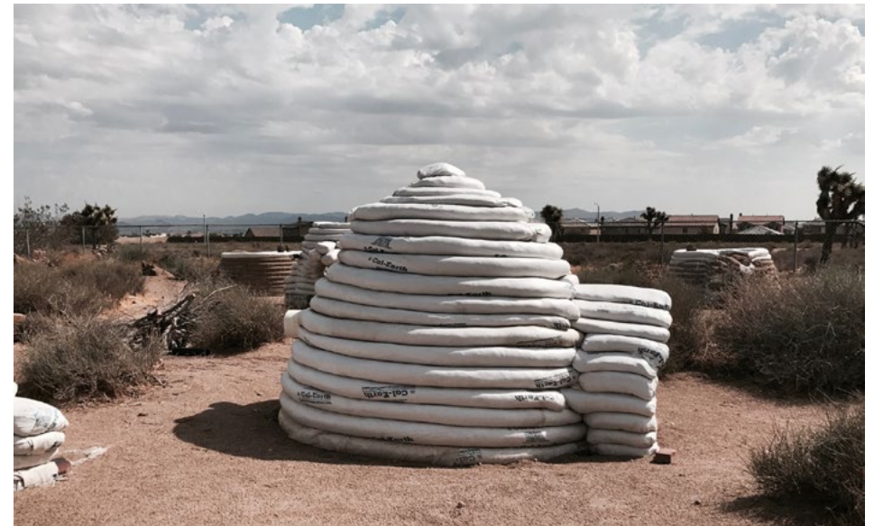
Cal Earth's technique of laying sacks of dry earth to form a domed structure was developed as disaster relief housing. This technique is very quick to learn and structurally robust.
