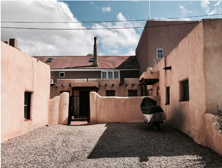
Houses in Taos made from low cost Adobe brick have become the most desirable and fashionable form of construction.
