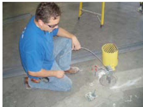
Electrician installing floor-mounted power outlets
