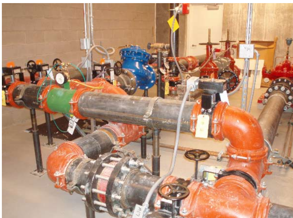
Southland Industry pipe installations at South Coast Hotel, Nevada
