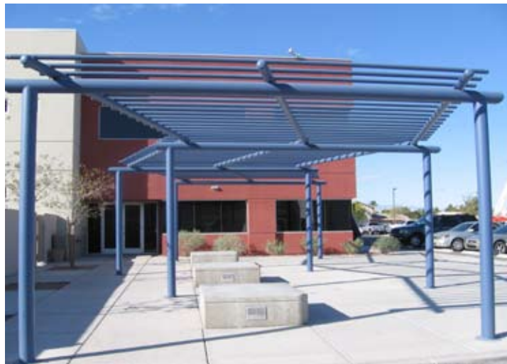
UA Local 525 apprentice-built pipe structure walkway
