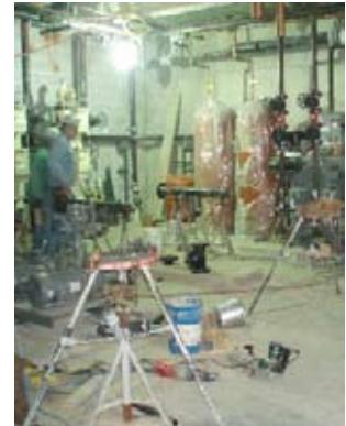
St. Joseph's Hospital pipefitting site construction
