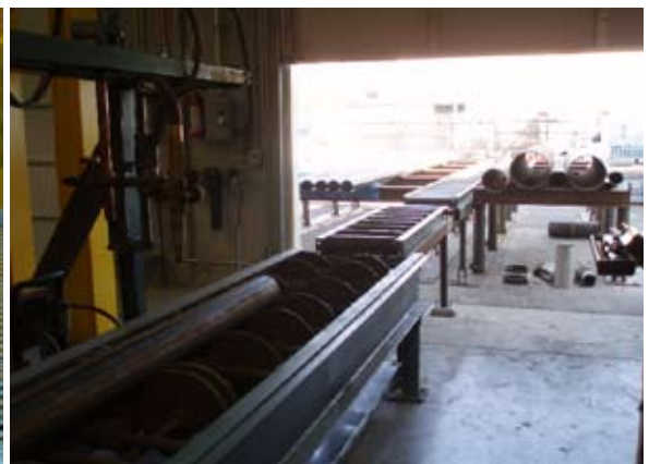
Pipe roller manual handling at Southland Industries
