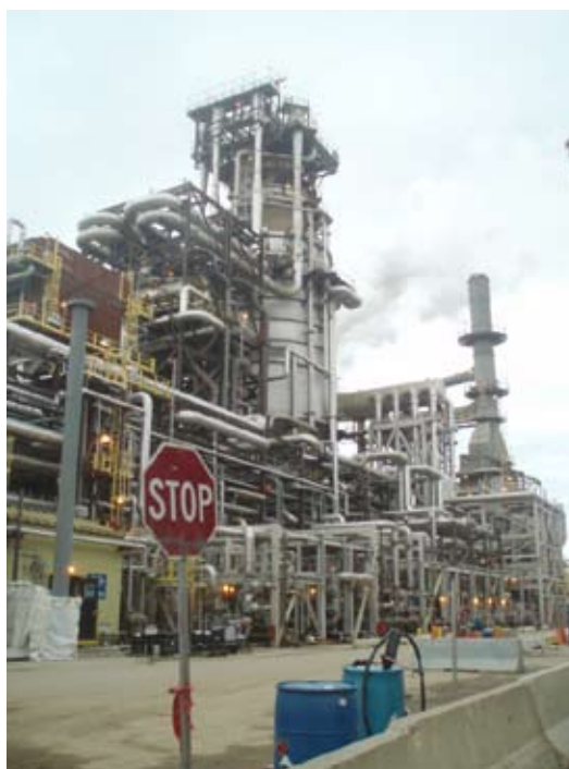
Piping at Syncrude Oil Refinery Fort McMurray Canada 2006 Image courtesy Syncrude Canada Ltd.
