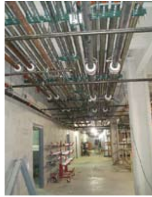
Pipefitting installations St. Joseph's Hospital Ann Arbor
