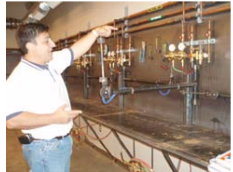
Phil Campbell in the medical gas welding workshop
