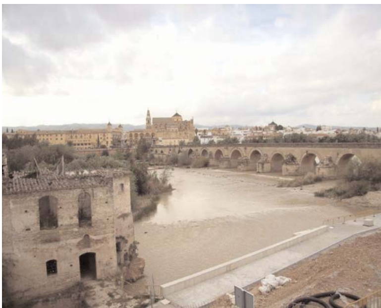
Left) Same location from the other side of the river. At the lower left is the remains of a water mill, one of a string on islands in the same river, below the Roman bridge. These mills both lifted water for the city's supply, and used its power to grind flour. In the foreground is a riverfront walkway under construction, in post-modern style, part of a program of urban renewal underway by the regional government.
