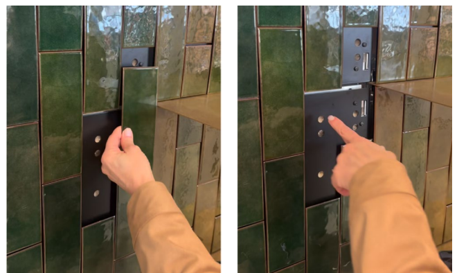
Figure 35. A Maniera tile being removed, showing the fastening mechanism that allows Incalmi's enamelled copper cladding system to be rearranged and reused rather than fixed permanently to a wall.
