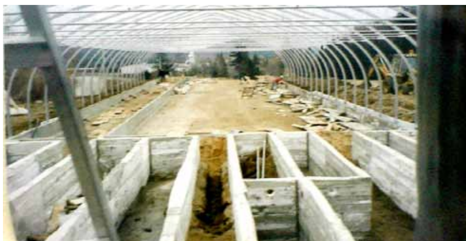
Concrete skeleton of production area
