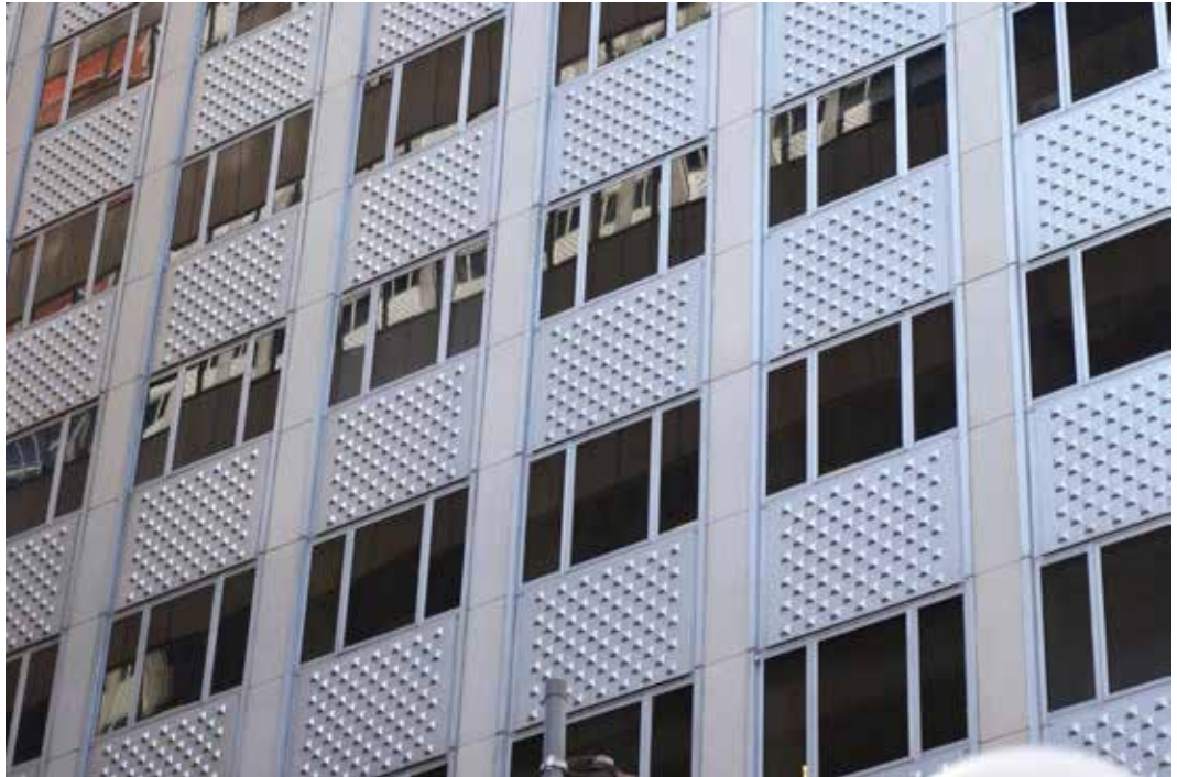
Figure 4: Aluminium façade of 666 Fifth Avenue, New York. Photo: Ruth Redden
