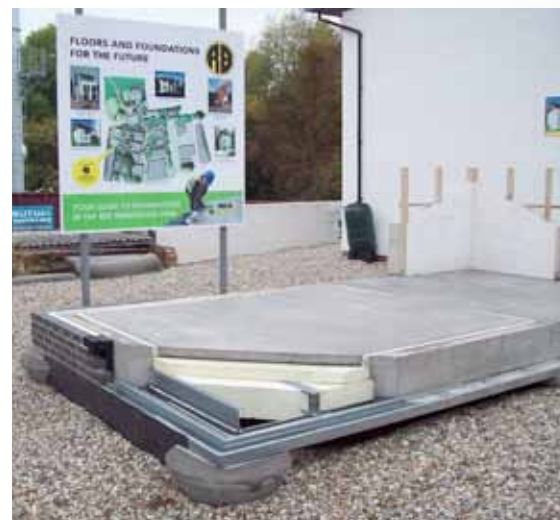
Figure 29: Insulation used as part of concrete raft slab construction (note the insulation is part of the slab)
