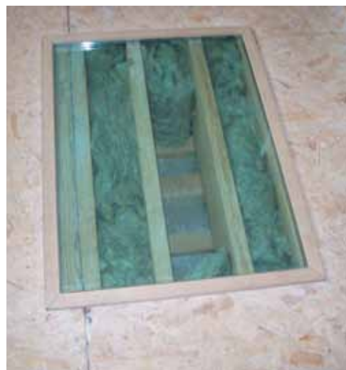
Figure 28: Insulation used to reduce heat loss between floors
