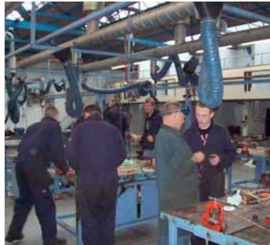
Figure 13: FAS plumbing teacher Brendan O'Reilly teaches apprentices copper brazing techniques, to help with their solar hot water installation skills
