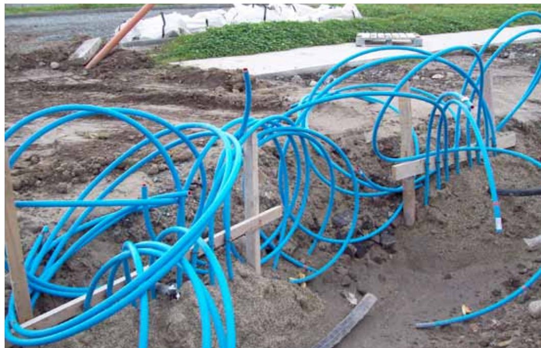
Figure 6: Flow and return collector poly pipe lines from lawn area (note: the lines are not yet connected to the manifolds).
