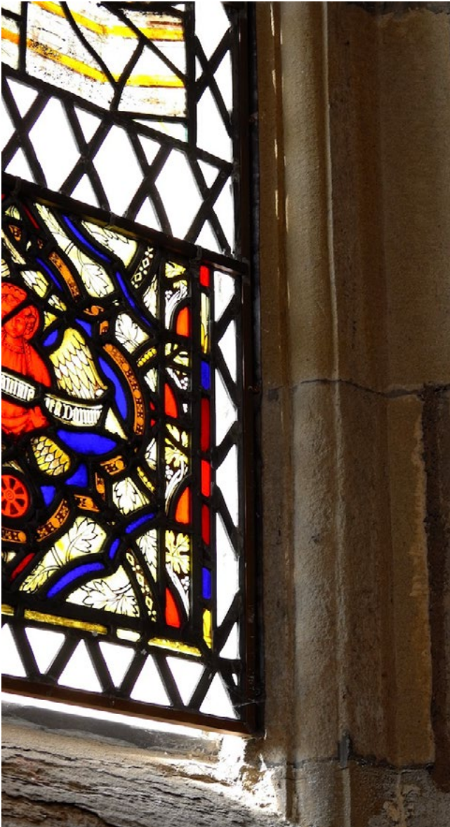
Figure 18. Image one: Internally ventilated EPG system
