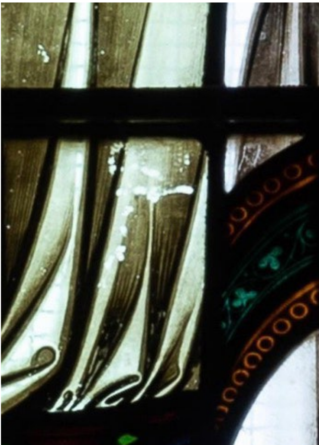
Figure 8. Image four: Paint loss detail from Ferguson and Urie detail from the tracery of St Paul's Anglican Church in Latrobe Terrace Geelong, made circa 1867. (Photos Courtesy of Ray Brown.)
