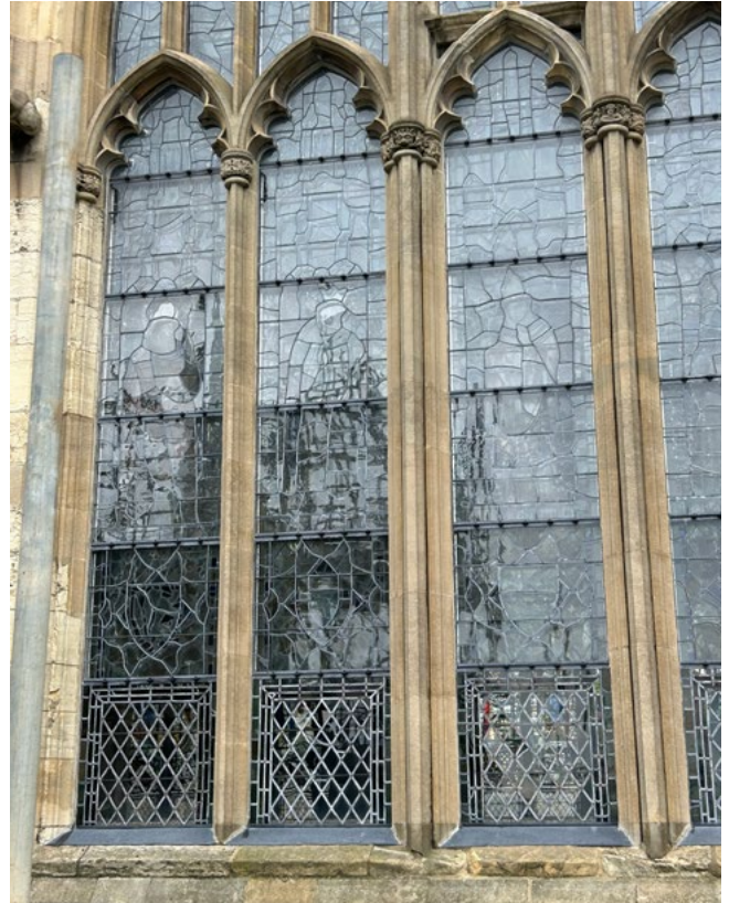
Figure 21. internally installed environmental protective glazing in-front of quarry leadlights, installed by Barley Studios.
