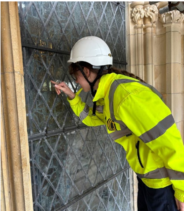
Figure 2. the Fellow on site at York Minster viewing Environmental Protective Glazing
