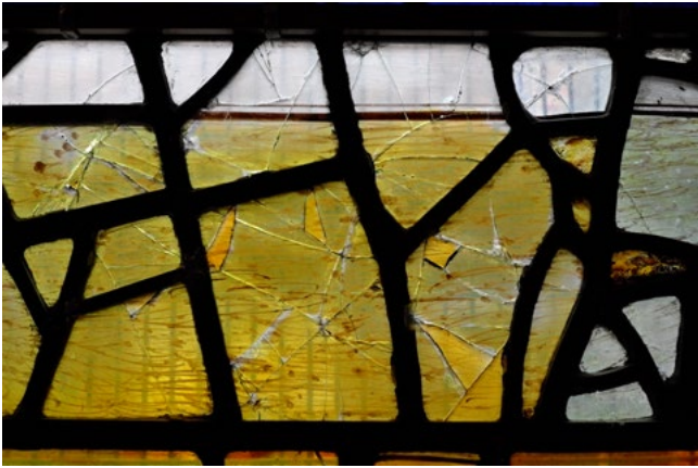
Figure 11. Edge Bonding at Merchant Taylors Hall, York.
