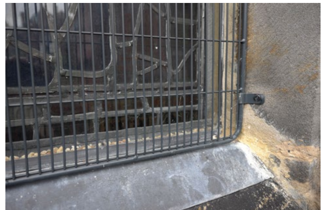
Figure 20. Lead upstand pictured in EPG system installed by Barley Studios.
