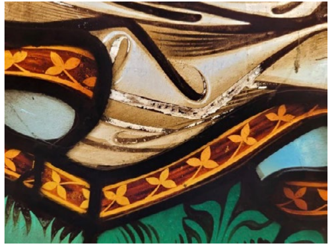
Figure 7. Image one, two and three: Paint loss detail from Hardman, Powell & Co, Great West Window in St Patrick's Cathedral, Melbourne. (Photos Courtesy of Bruce Hutton, Almond Glassworks.)
