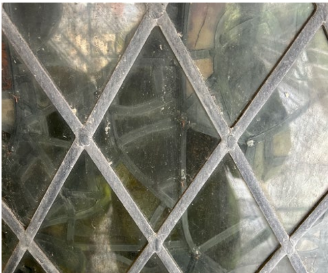
Figure 22. Historical stained glass environmental protective glazing with quarries on York Minster.
