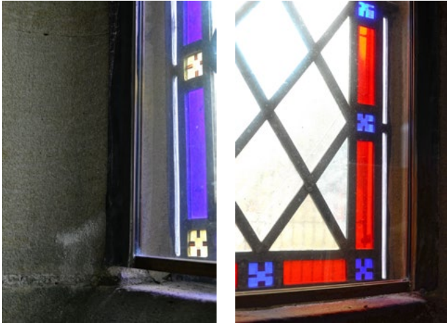
Figure 21. internally installed environmental protective glazing in-front of quarry leadlights, installed by Barley Studios.
