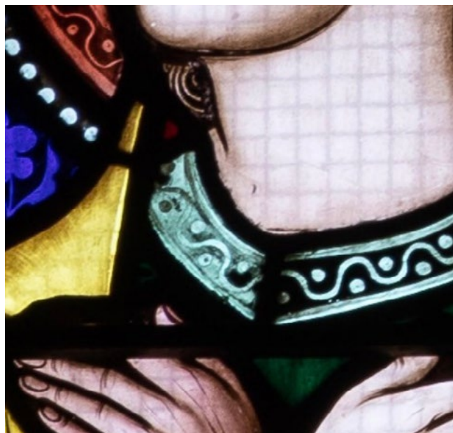
Figure 10. Image one: Paint loss detail from Hardman, Powell & Co, Great West Window in St Patrick's Cathedral, Melbourne. (Photo Courtesy of Bruce Hutton, Almond Glassworks)
