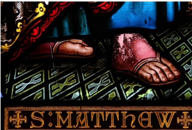
Figure 9. Image five and six: Paint loss detail from Ferguson and Urie detail from All Saints Anglican in South Hobart , made circa 1868. (Photos Courtesy of Ray Brown.)
