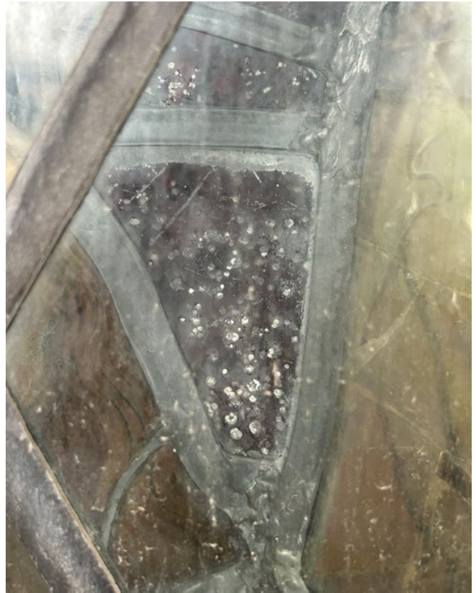
Figure 14. Medieval glass corrosion at York Minster
