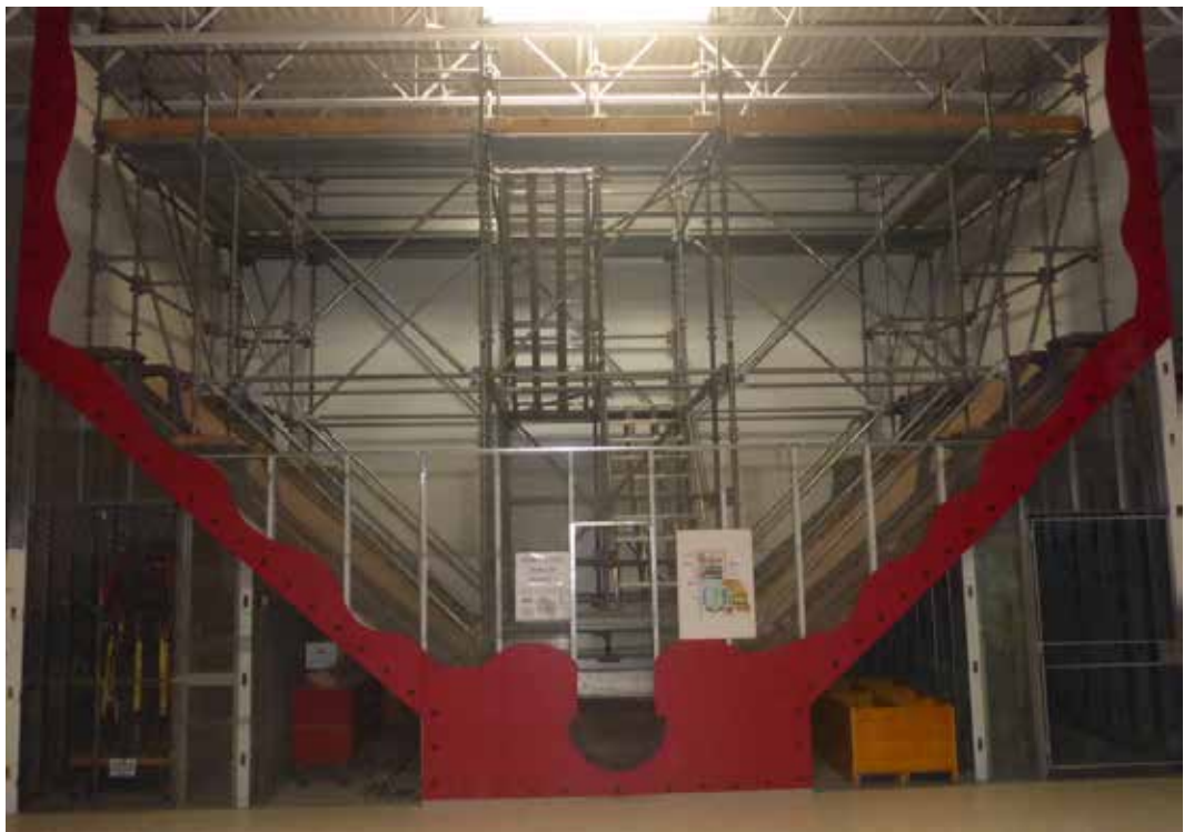
Multi level scaffolding project and assessment
