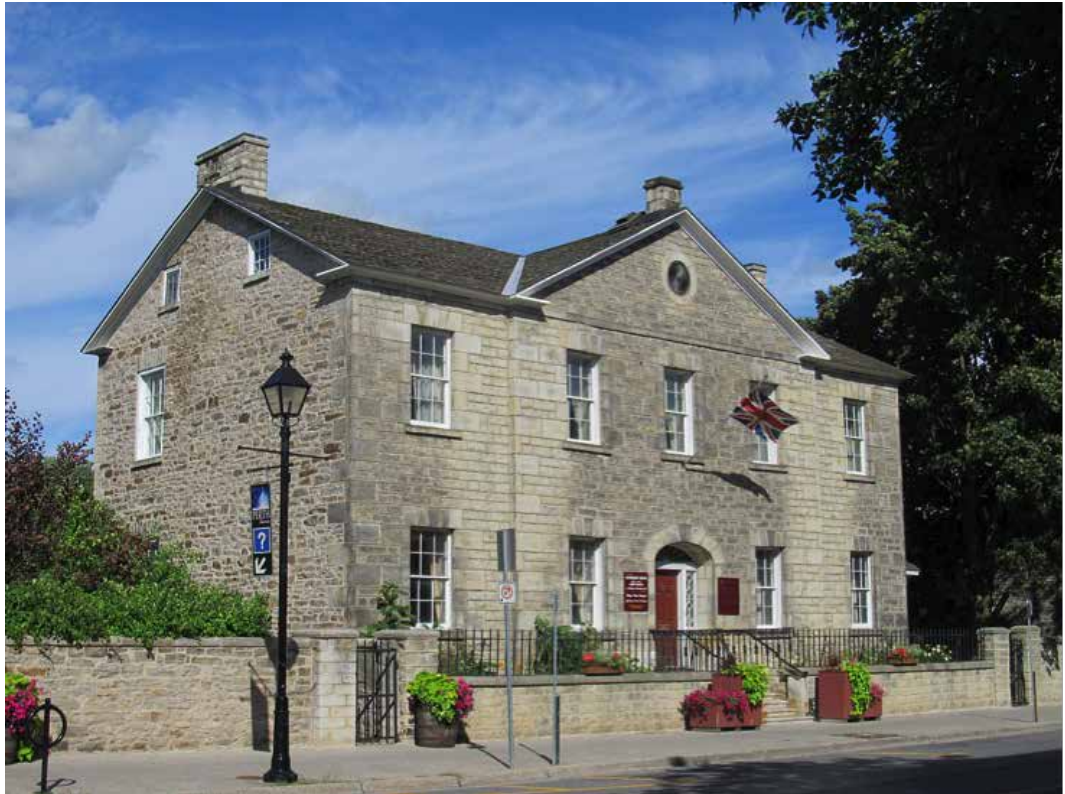
Matheson House ,Perth Ontario National Historic Site and local museum. Window restoration by Algonquin carpenters
