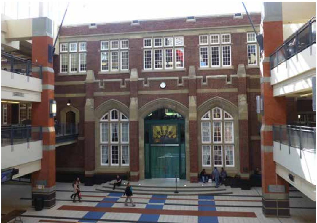
SAIT Original Heritage Building
