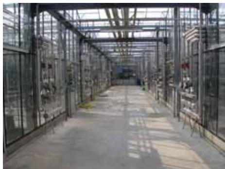
Entrance to PTC+ glasshouse facility
