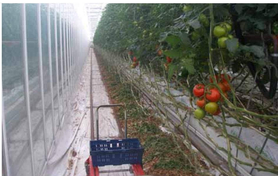
Hanging gutter system and heating pipe/rails
