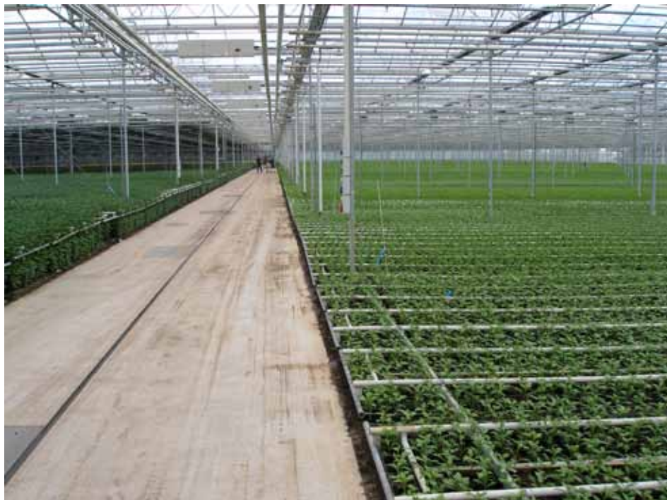
Main glasshouse unit
