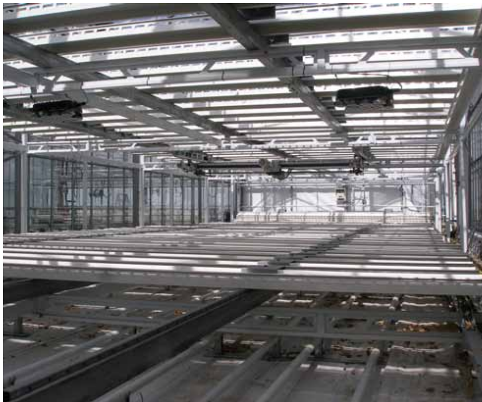
Automated pot plant gutter system
