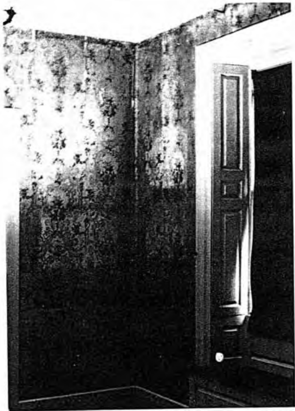
FIG. 3 Parlor paper before treatment. Heavy dirt and soot accumulation. Design loss from furniture abrasion at lower left.
